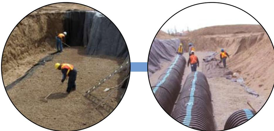
Engineers from Pitura Husson approved the CULTEC system which consisted of 1,380 Recharger® 330 HD chambers configured in eight storage beds. The Recharger chambers are dome-shaped with perforated sidewalls and fully open bottoms to allow for maximum infiltration. In addition, placed at the front of the system were nine CULTEC
